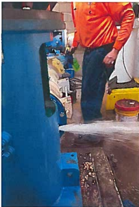
Initial activating pump motor. A plug was removed to prevent high pressure from blowing out gaskets, CLA-VAL, and other water components.
