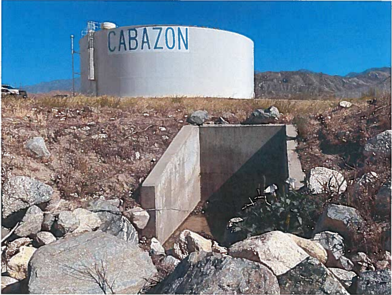
Overflow discharge from T1
