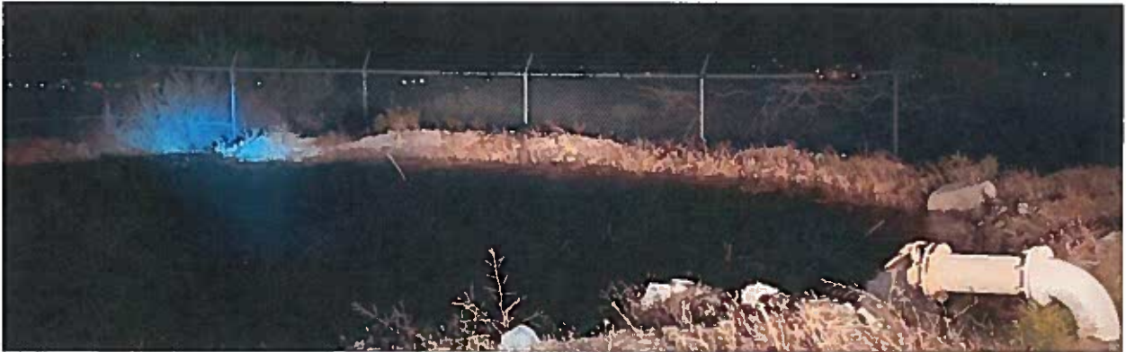
As planned, waste water pond overflow is being discharged out into the field.
